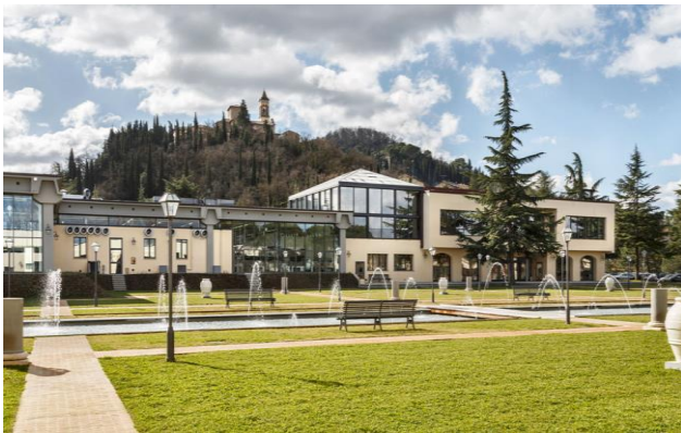
Figure 13 – Exterior View of the Solomeo Industrial Park 61
